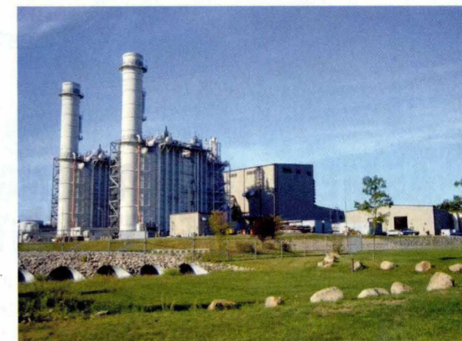
The 550-MW Rhode Island State Energy Center in Johnston is one of the efficient combined cycle gas turbine power plants that replaced coal power in New England.
